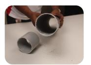
Before applying solvent cement, insert the pipe end into the socket of the next pipe or fitting to check that interference occurs at about 1/3 to 2/3 of the socket depth.
