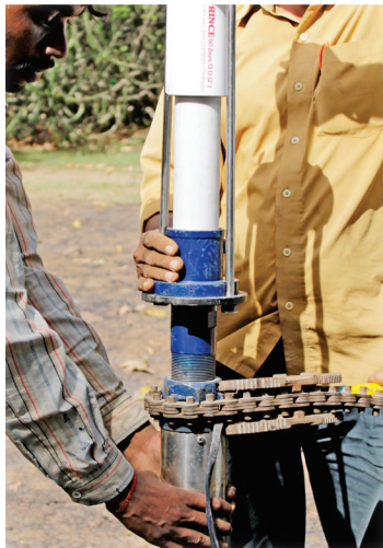
Before joining the pipe with the pump, ensure pump guard is installed properly.
