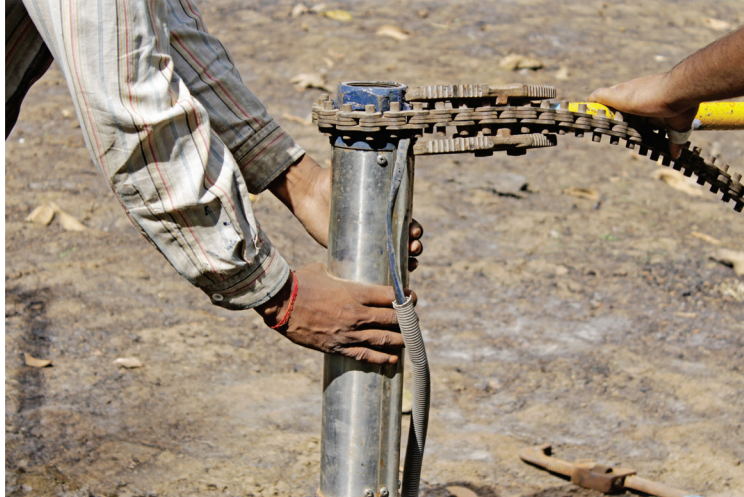
Join Metal connector to submersible pipe with the help of chain wrench.
