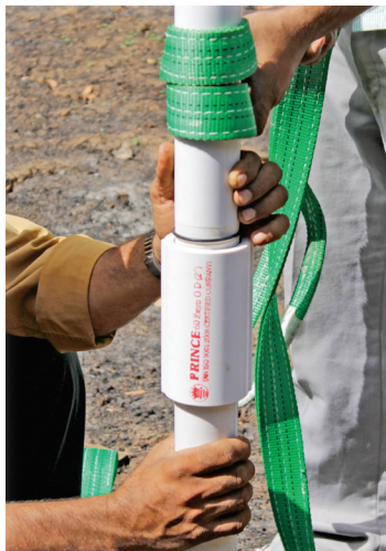
Tighten pipe till half rubber ring is seen with hand, if required use belt wrench for final jerk.
