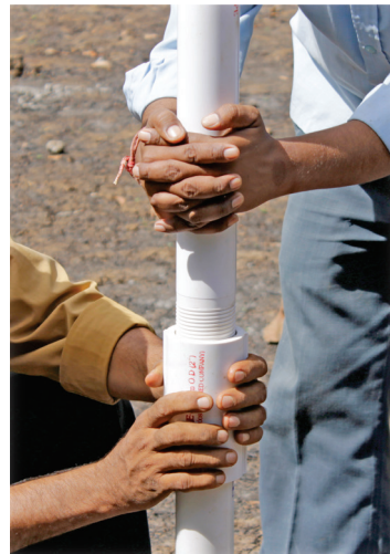
Before opening or joining the pipe, ensure the coupler is firmly held by the hand.
