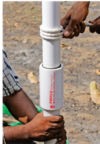
Tighten pipe till half rubber ring is seen with hand. If required use rope wrench to give a final jerk.
