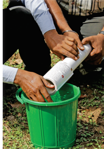
Before starting pipe assembly clean the pipe threads with clean water.
