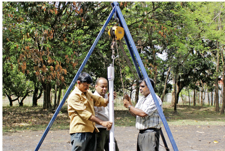
Lower SUBMERSIBLE DELIVERY PIPE with the help of a chain pulley.
