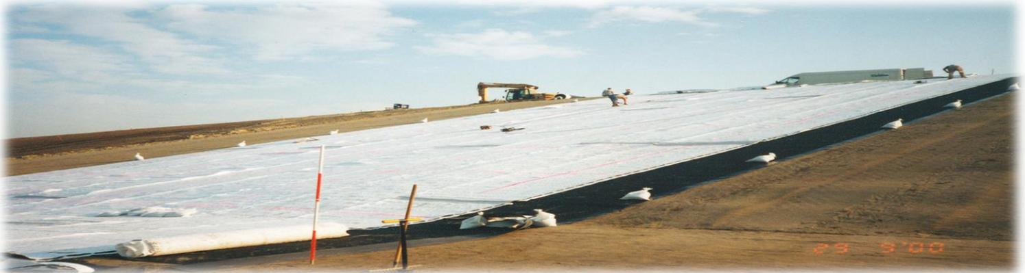
Roads RE Wall , Levelling and mechanical protection of the geomembrane; drainage of the accidental leaks below primary ; leachate and rain water collection above primary geomembrane; mechanical protection of the geomembranes when in contact with waste-materials and/or soil; drainage of liquids and gases present in the soil above and/or below the capping geomembrane.
