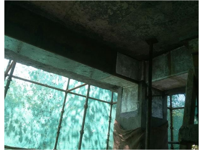
FIBER WRAPPING TO BEAM & COLUMN
