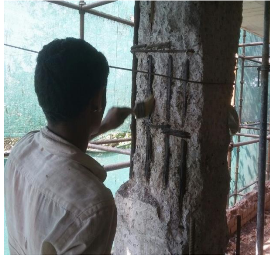
REINFORCEMENT TREATMENT
