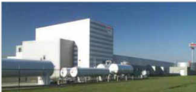
Soudal PU foam production: Turnhout, Belgium
