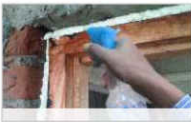
Spray some additional water on applied PU foam on both sides of the door frame.
