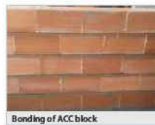
Bonding of ACC block
