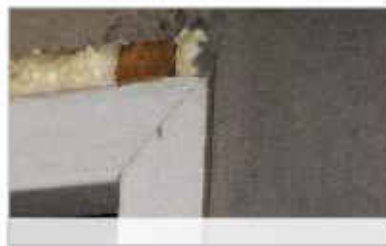
After curing PU foam can be plastered or covered with architrave/moulding.
