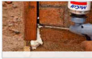
Hold the PU foam can upside down & extrude the foam by pressing the bar/application gun.
