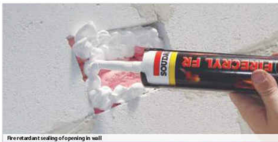
Fire retardant sealing of opening in wall
