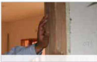
Do not touch the frame during curing of the PU foam otherwise you will break the cell structure and the adhesion will be lost.
