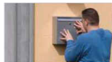
Bonding of all materials (interior & exterior)
