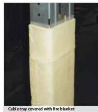
Cable tray covered with fire blanket
