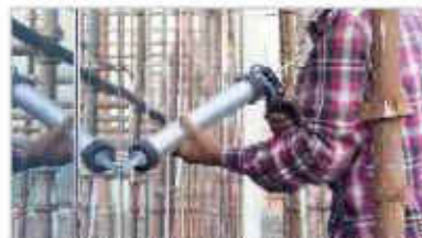
Silirub 989 & Silirub WSL+ sausage application
