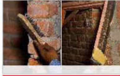
Surface needs to be clean, dust-free, free of oil & grease.
