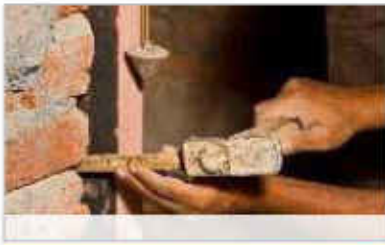
Align your door frame and block it with wooden blocks between frame & wall.
