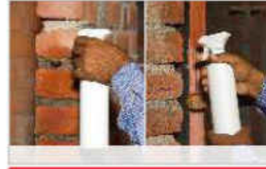
Slightly humidify the surface & the door frame before applying the foam.
