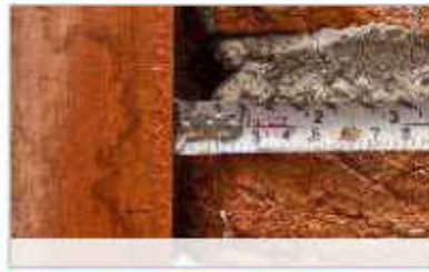
Keep a gap of 10 mm to 20 mm between wall and door frame on the three sides of the frame.
