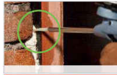
Small gaps (less than 5-7 mm) can be filled by using plastic extension which comes with every application gun.
