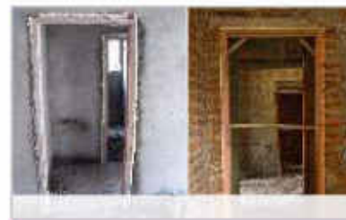
Perfect installed door frame with PU foam.
