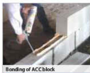
Bonding of ACC block
