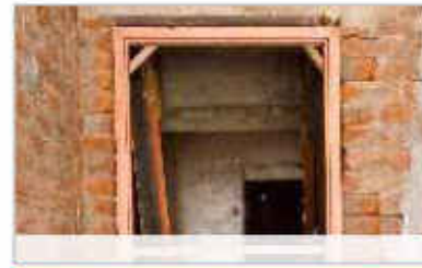
Aligned door frame.
