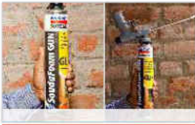
Shake the PU foam can minimum 20 times before application to obtain the best PU foam quality.
