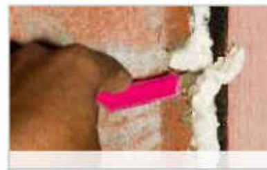
Cut the spoiled foam at the time of plastering.
