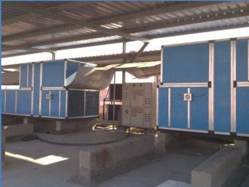
Air Handling Unit With Heat Recovery Wheel & Electrical Heaters
