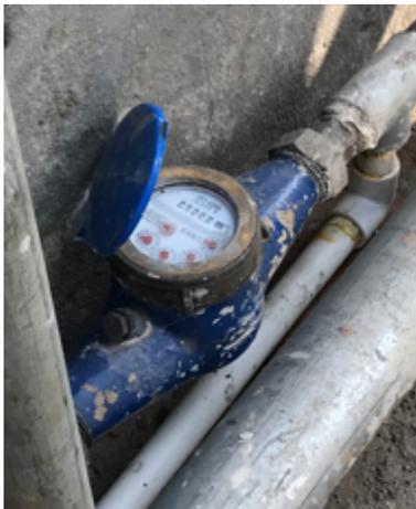
Figure 3: Water flow meter for measurement of input water
