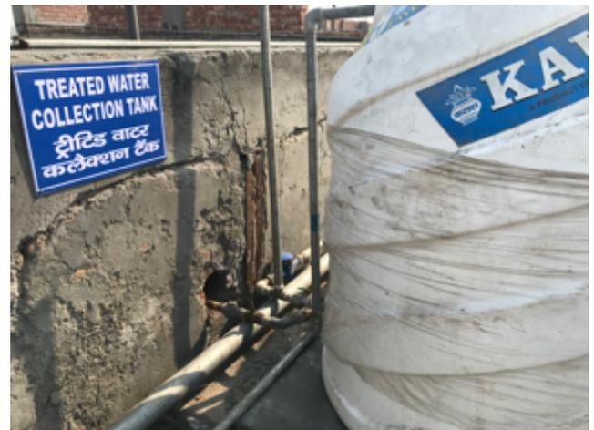
Figure 4: Tank for treated effluent after ultrafiltration
