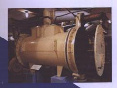
These condensers are heat exchangers which convert steam from its gaseous to its liquid state at a pressure below atmospheric pressure. the purpose of a surface condenser is to condense the exhaust steam and convert the exhaust steam into pure water so that it may be reused in the steam generator or boiler as boiler feed water.
