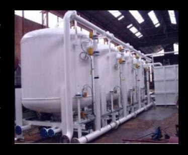
Pressure Sand Filter Typically used for removal of suspended solids & undissolved impurities like dust particles & heavy metals etc. doing so it reduces turbidity. Sand filtration is used for cooling water, treatment of Wastewater and filtration of surface water.
