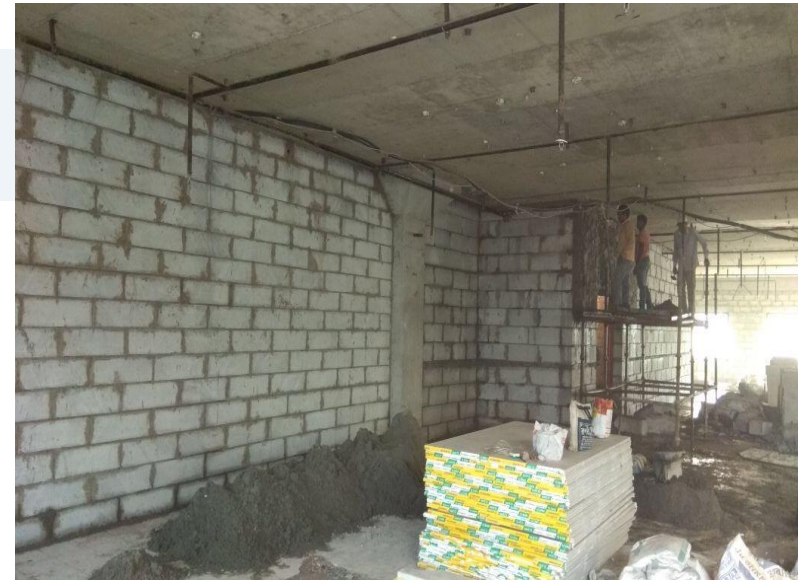
Civil work at vatika first india place
