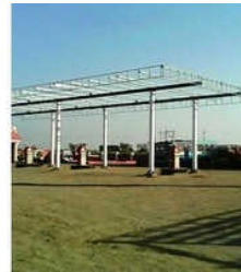
Prefabricated Petrol Pump Structure
