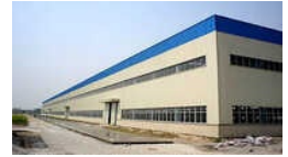
MS Prefabricated Building
