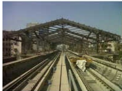
Prefabricated Metro Stations Structure
