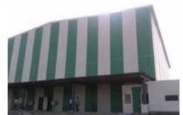
Prefab Cold Storage Room
