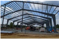
Prefabricated Industrial Structure
