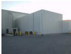
Industrial Cold Room
