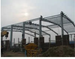
Pre Engineered Building Structure
