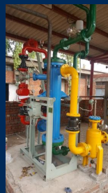
Industrial Gas Pipeline Fitting
