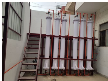
Gas Pipeline Fitting
