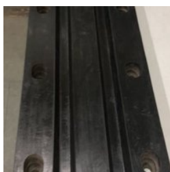
Slab Seal Expansion Joint
