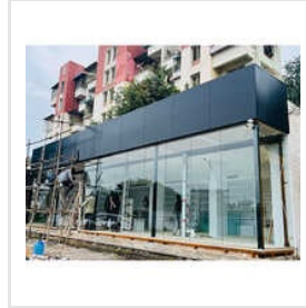
Commercial Glass Partition
