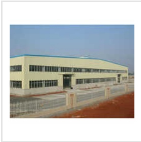
Heavy Steel Structures Fabrication Service
