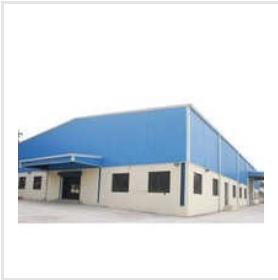
Industrial Shed Fabrication
