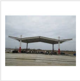
Toll Plaza Canopy
