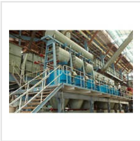
Sugar Mill Fabrication Service
