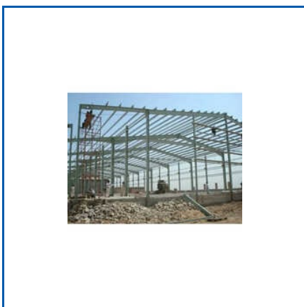
INDUSTRIAL SHED FABRICATION SERVICE
