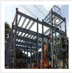
Heavy Industrial Fabricator Service
