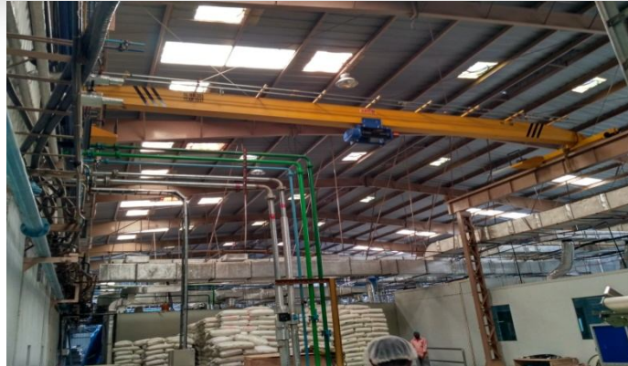
Customer: Manjushree Technopack Limited 1Ton Capacity Single Box Girder EOT Crane
