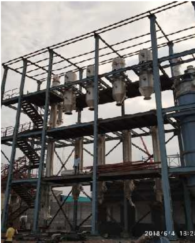
Sadekar Enviro Engineers plant under Erection and Commissioning
