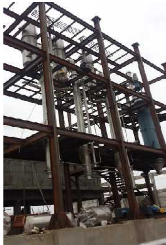
Agrisol India Pvt. Ltd plant under Erection and Commissioning
