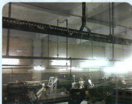
FOGGING SYSTEM FOR COTTON WEAVING
