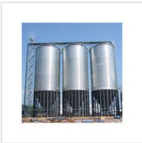
Hopper Bottom Silos
