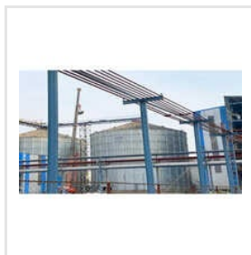
Grain Storage Silos System
