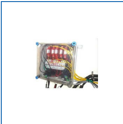
DEHN SURGE PROTECTION DEVICE
