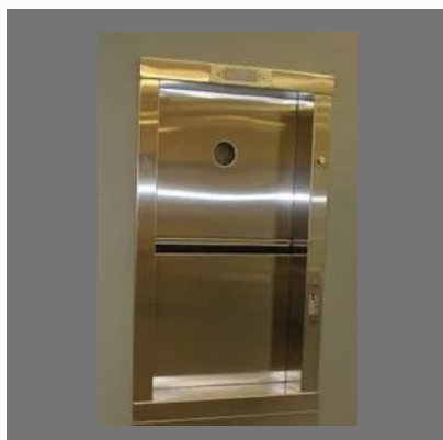
Dumbwaiter Service Lifts
