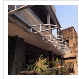
Industrial MS Structure
