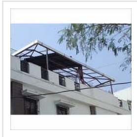
MS Roof Shed Structure
