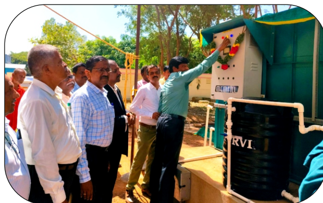
HyBRIT STP Plant Inaugurated by Dr.Ravi, Vice Chancellor at Alagappa University
