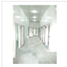
1500 MT Multipurpose Cold Storage
