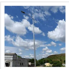
High Mast Lightning Pole
