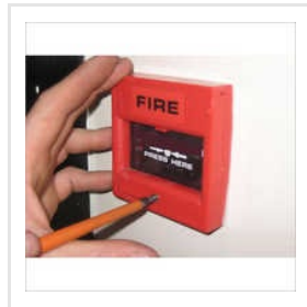
Fire Alarm Installation Service
