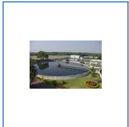
COMMERCIAL SEWAGE TREATMENT PLANT
