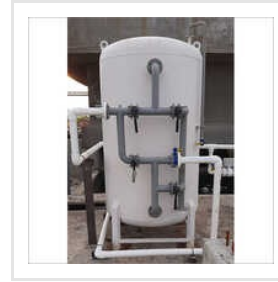
Pressure Sand Filter
