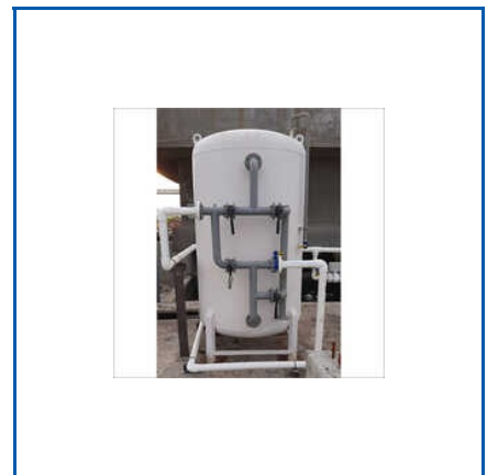
PRESSURE SAND FILTER
