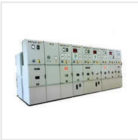
Industrial MV Panel
