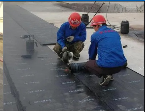
Roof Membrane Waterproofing Service
