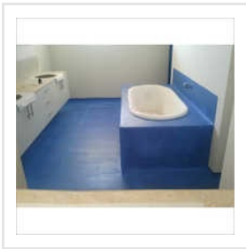
Toilet - Bathroom Waterproofing Service
