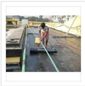
Bituminous Waterproofing Service
