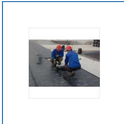
ROOF MEMBRANE WATERPROOFING SERVICE
