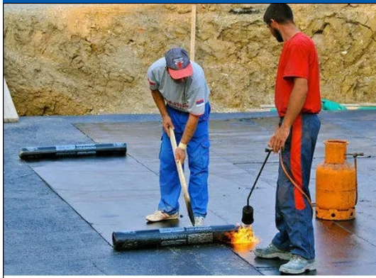
APP Bituminous Membrane Waterproofing Service
