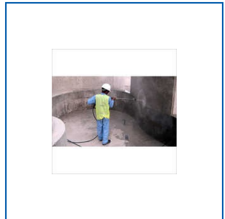
WATER TANK CRYSTALLINE WATERPROOFING SERVICE
