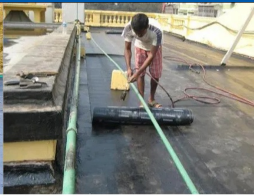
Bituminous Waterproofing Service
