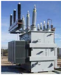
Electrical Power Transformer
