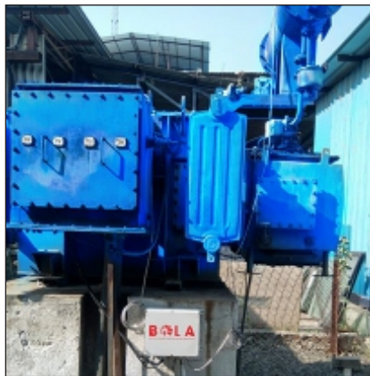
Power Distribution Transformer
