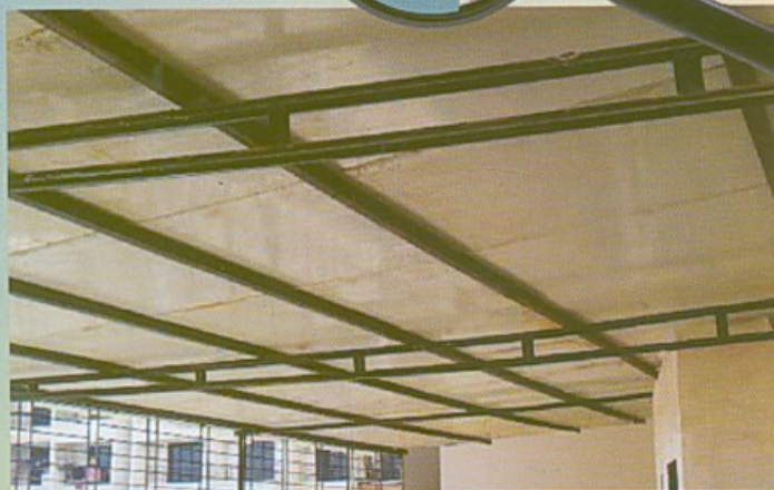
Internal View After Fixing PUF Insulated Panels
