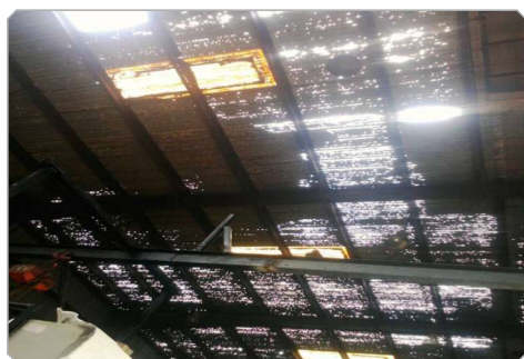
OLD CORRODED ROOF (METAL)
