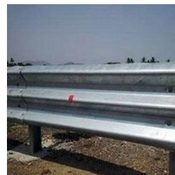
Thrie Beam Barrier
