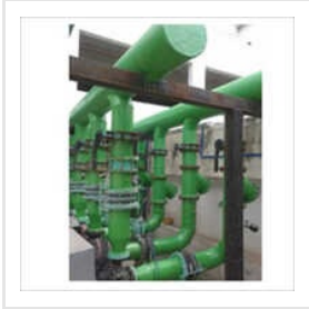
FRP Lining Of MS Pipeline
