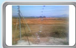
Solar Power Fence
