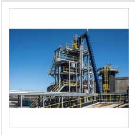
Gas Recovery Plant Structure Fabrication
