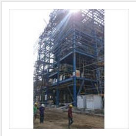
Steel Structural Erection Services
