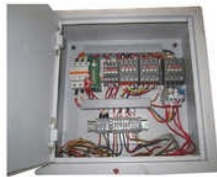
Three Phase Control Panel
