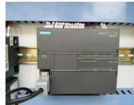
SIEMENS PLC Control System
