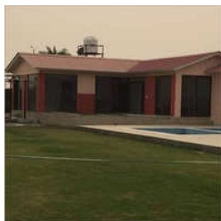
Prefabricated Modular House
