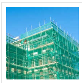
Construction Safety Net
