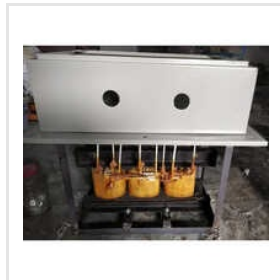
60KVA Step Down Transformer
