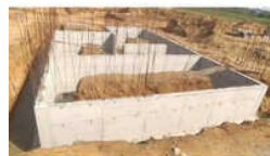
Concrete Formwork Shuttering
