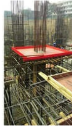
Nova Formwork Slab Formwork
