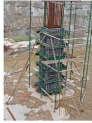
Concrete Wall Formwork
