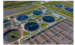
Industrial Effluent Treatment Plant
