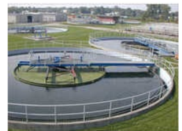
Industrial Water Treatment Plant
