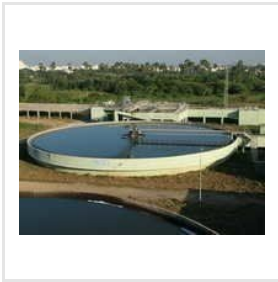
Circular Mechanical Clarifiers
