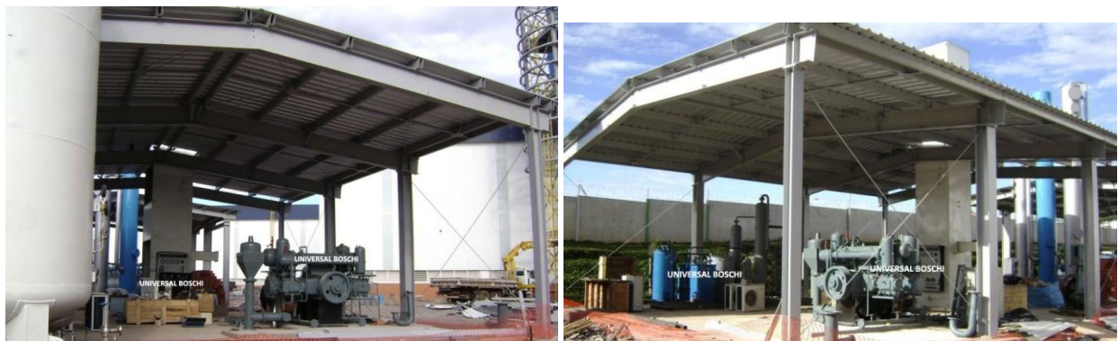
Erection of UBL 150 at Metasa Steel Plant in Brazil
