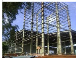
Foundries Steel Structure Building
