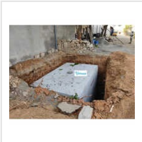
Sewage Water Treatment Plant
