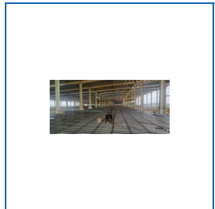
SHEAR STUD WELDING /FIXING SERVICES
