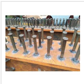
Shear Stud Welding Job Work
